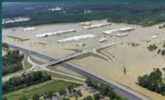
Juban Crossing at Peak of Flood Interstate 12 at Juban with Flood Water Level with Center Barrier Wall
