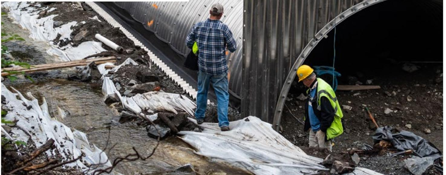
Peterson Creek flows through a temporary channel (left) while the new fish-friendly arch culvert was installed.
