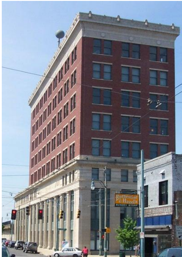
Figure 11: Restored Central Station
