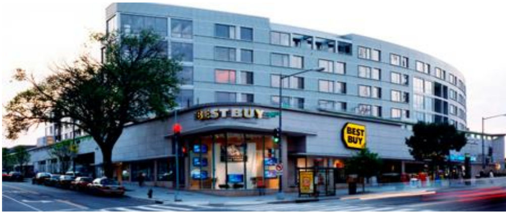
Figure 13: Historic Sears Roebuck Store with Condos Built Atop Existing Parking Deck
