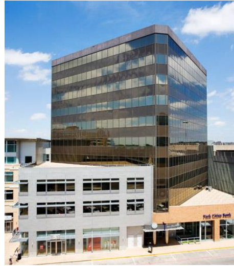
Figure 27: Office Building at Mockingbird Station
