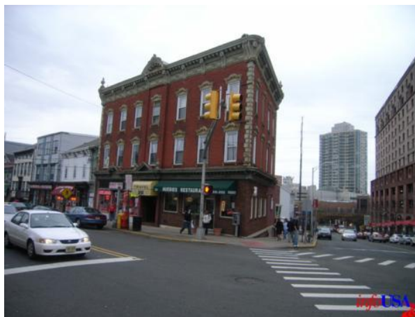
Figure 19: Portion of Gateway Transit Village Site, on Somerset Street: Before Development
